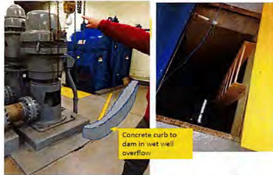
Photo 3: Gander Lakeside wet well curbing
