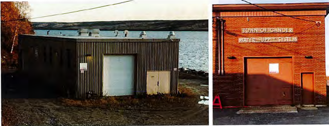
Photo 1: Gander Lakeside (left) and Reservoir (right) Pumphouses
