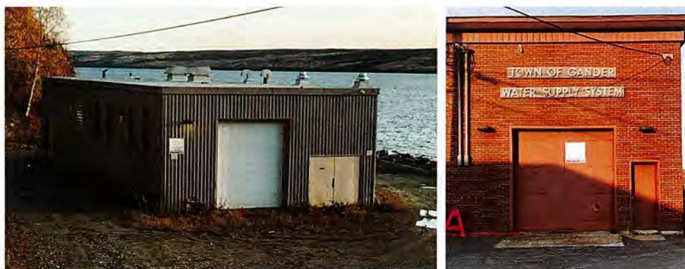
Photo 1: Gander Lakeside (left) and Reservoir (right) Pumphouses
